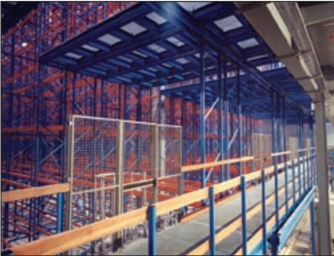
Mezzanine construction at the P&D-stations
