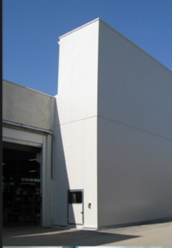
EXTERNAL UNICO external warehouse featuring internal bays
