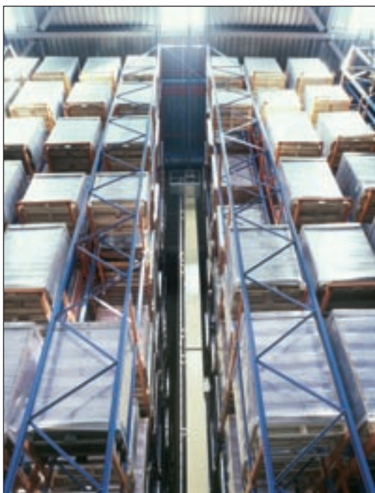
Aisle equipment: top ties, top rail and run-out construction
